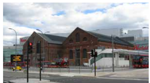
C DIMCO building
