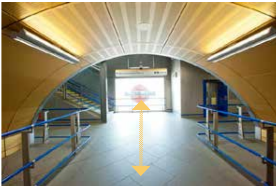
Figure 3.34: Potential provision for an additional entrance at Wood Lane Station Source: TFL
