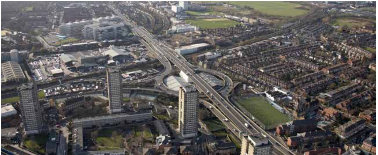
Figure 3.57 Aerial view of the Westway - existing
