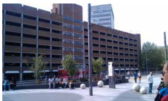
Figure 4.12: Existing public realm around DIMCO
