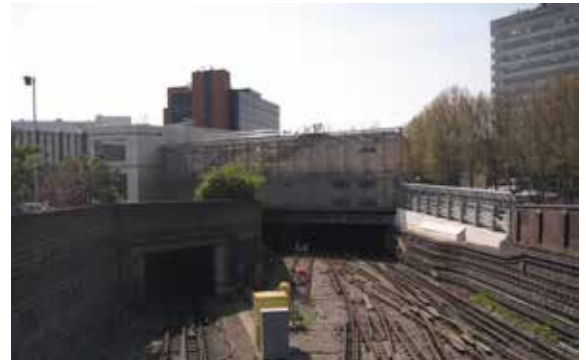
② Central Line cutting
