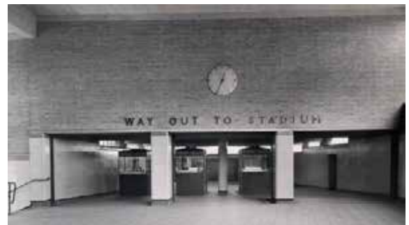
③ White City LUL Station, Central Line
