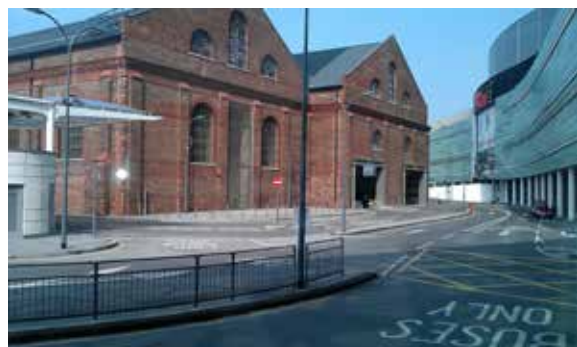
Figure 4.11: Existing public realm around DIMCO
