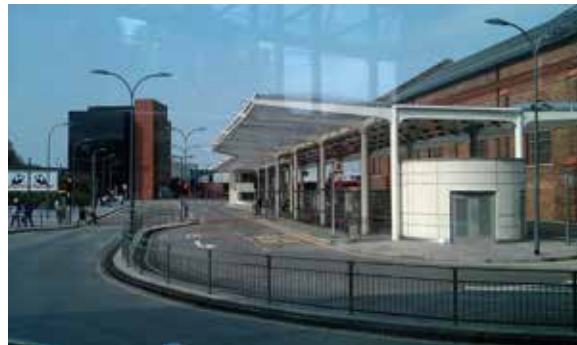
Figure 4.10: Existing public realm around DIMCO
