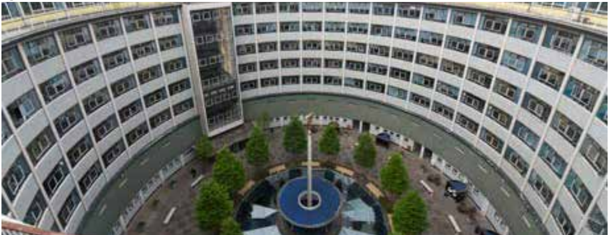
Figure 3.41: BBC TV Centre, Inner courtyard
