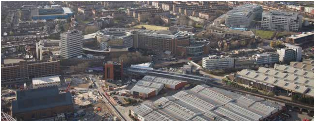
Figure 3.66: Aerial view of BBC TV Centre and the existing tower
