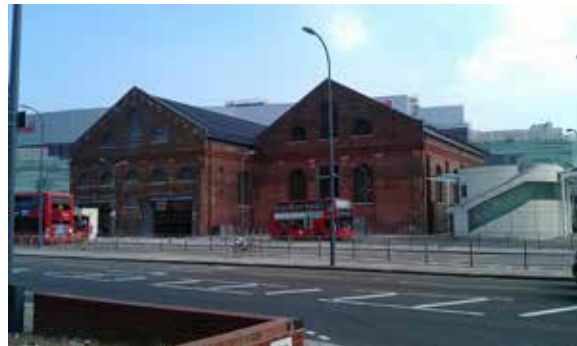
Figure 4.9: Existing public realm around DIMCO
