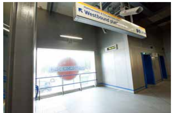
Figure 4.7: Potential Step-free access at Wood Lane
