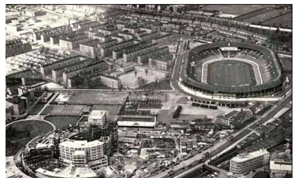
④ BBC TV Centre under construction
